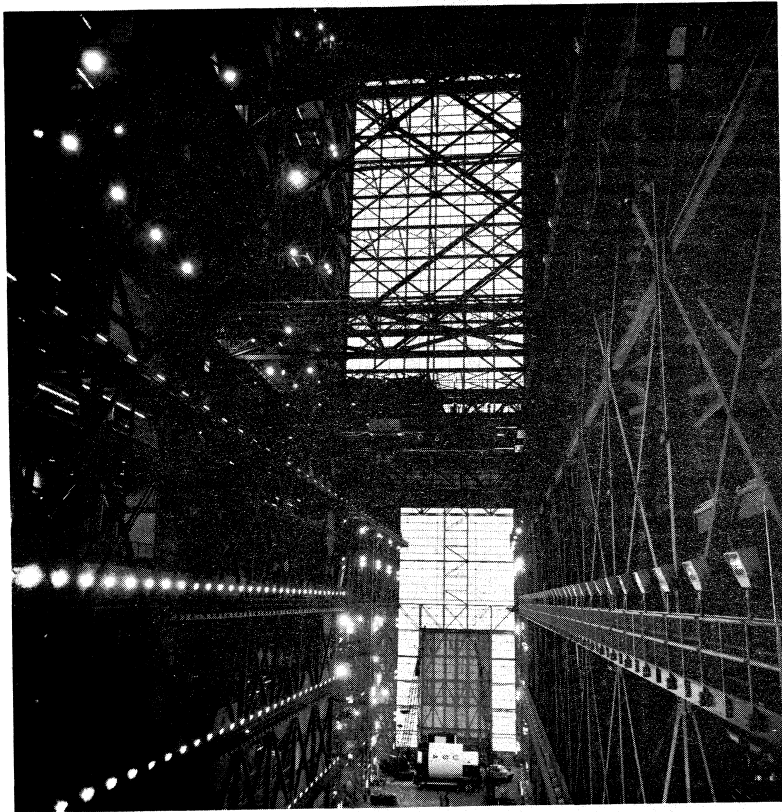
Interior view of transfer aisle, Vehicle Assembly Building, looking from High Bay into Low Bay.
