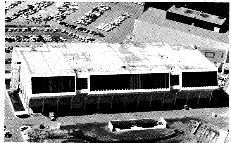
Launch Control Center in completed form showing window louvers.
