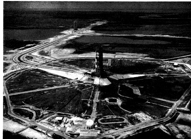
Aerial view of Launch Pad A showing Apollo-Saturn V and Mobile Launcher on pad. High Pressure Gas Storage Facility can be seen beneath hardstand, with liquid oxygen and liquid hydrogen storage tanks on far and near side of pad area respectively. RP-1 facility is adjacent to that for liquid hydrogen.
