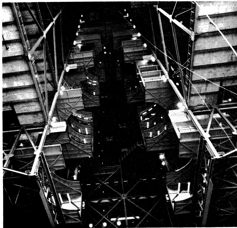
Extensible work platforms in High Bay 1, Vehicle Assembly Building, with upper platform closed, others in retracted positions.
