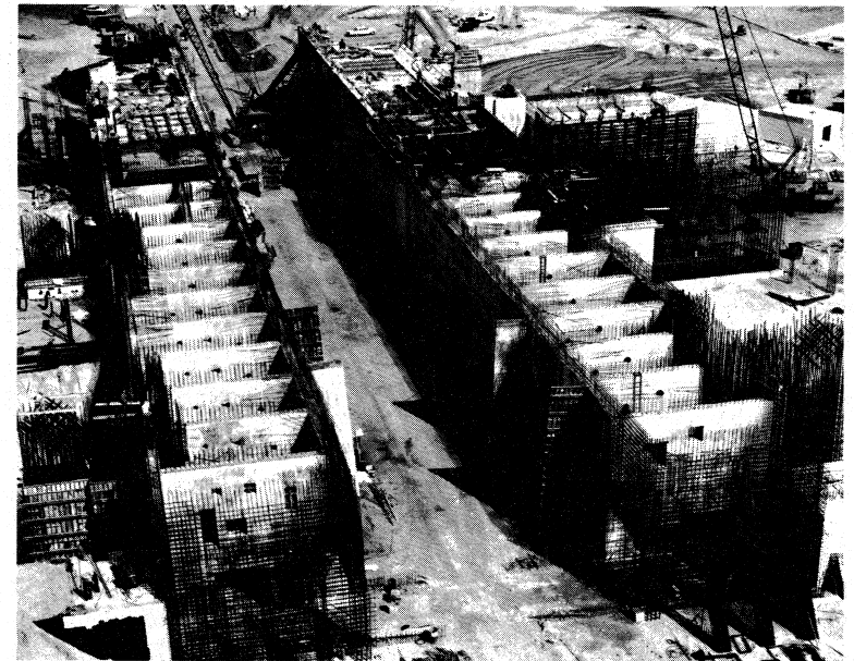
Cellular structures lining flame trench at Launch Pad B.
