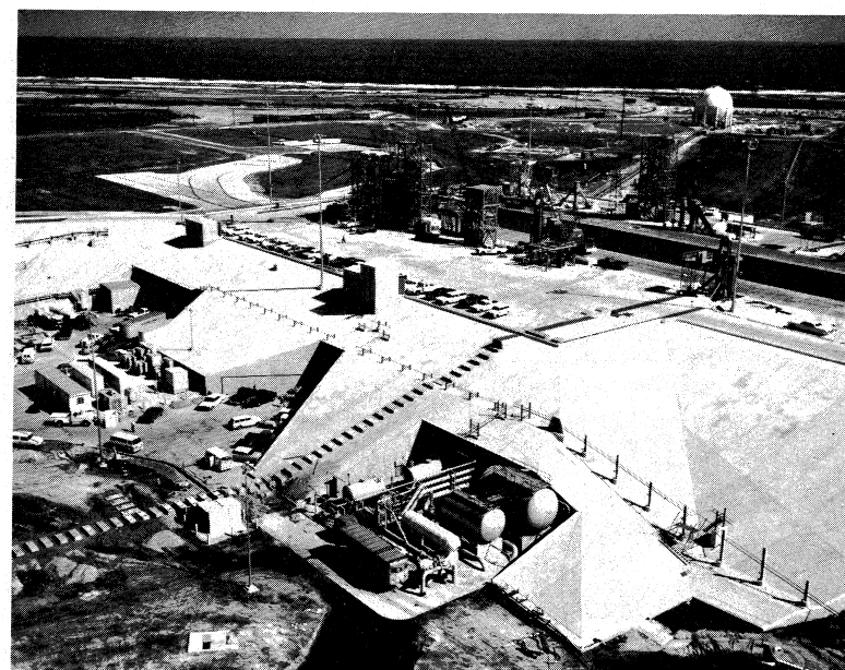
Launch Pad A hardstand area showing pedestals and service towers along with ground level entrances to Pad Terminal Connection Room (PTCR) and Environmental Control System (ECS) Room on near side of pad.
