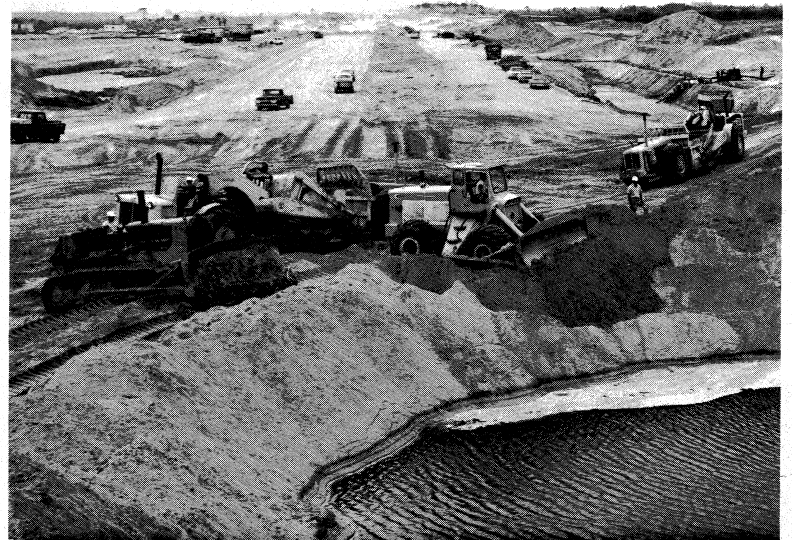
Placement of sub-base material in early stages of Crawlerway construction.
