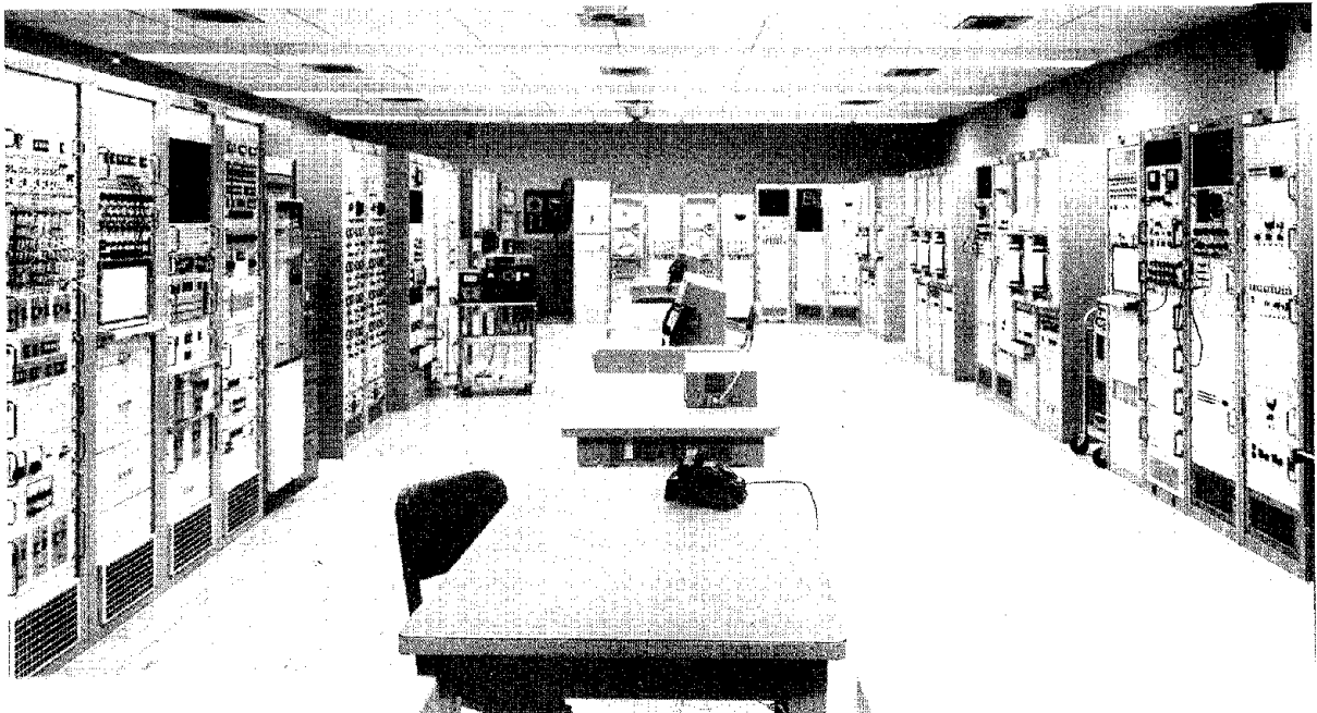
Figure 9-5. Instrumentation control center (VIB).
