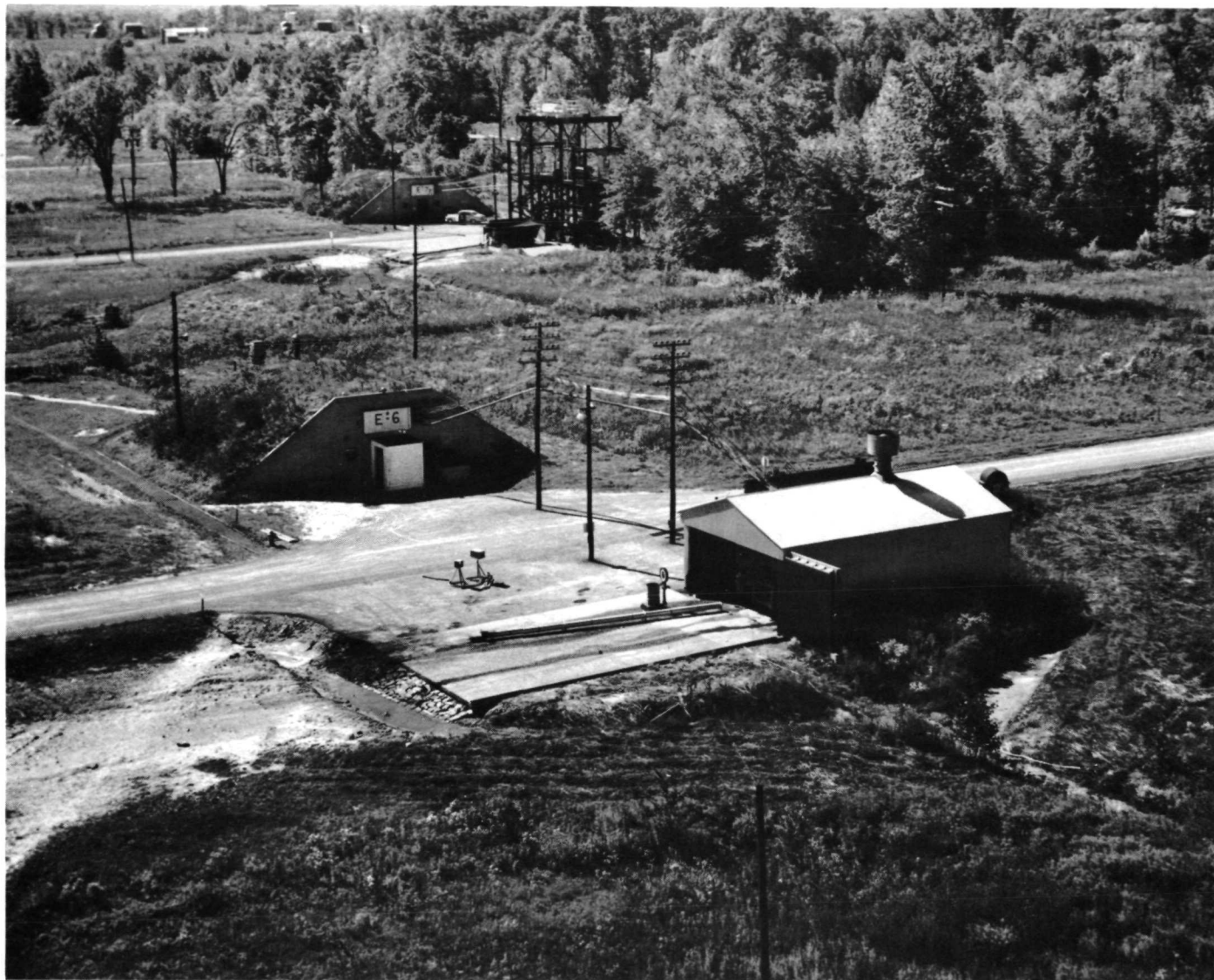
Figure AII-3. Test Stand and Instrument Control Room
