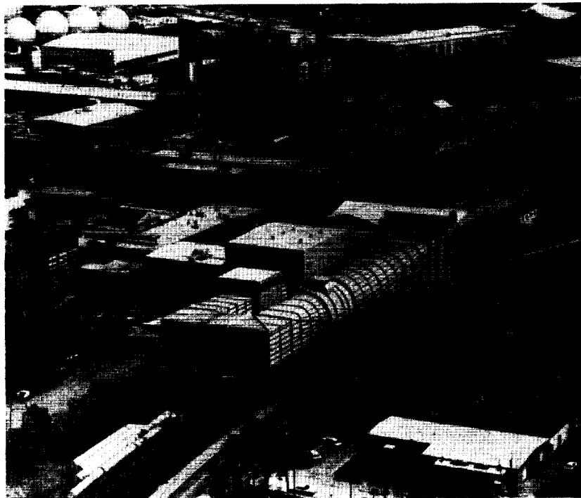
The Langley 14-by-22-Ft Subsonic Tunnel (formerly the 4-by-7-Meter Tunnel) is used for low-speed testing of powered and unpowered models of various fixed- and rotary wing civil and military aircraft. The tunnel is powered by an 8000-hp electrical drive system.
